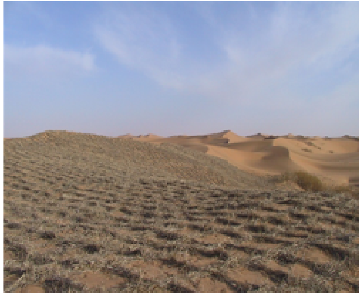
[Figure 7] The sand barriers of straw checkerboards
